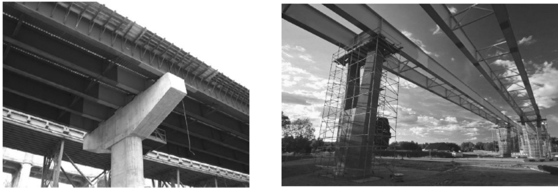
Figure 2.2 Bridges designed with hybrid steel plate girders.
