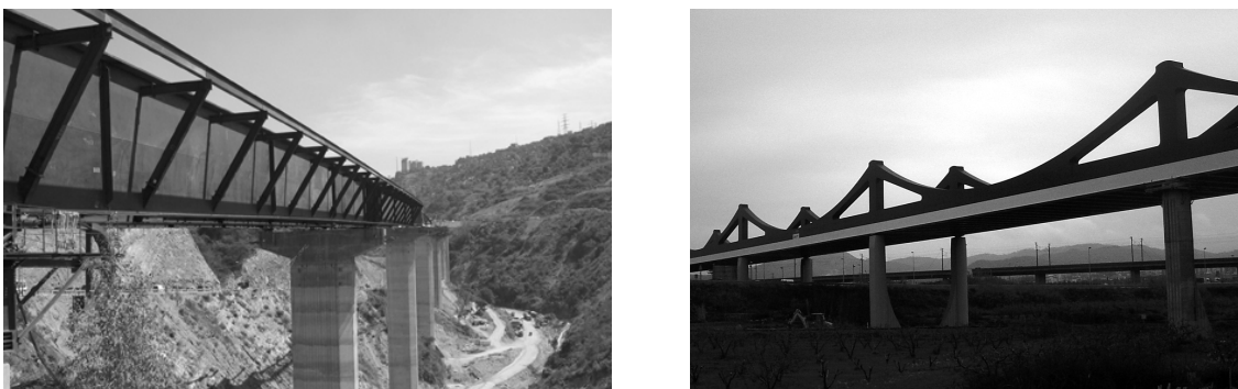
Figure 2.1. Girders in medium-span launched bridges. (a)Caracas-La Guaira Viaduct. Venezuela. (b) Sant Boi Viaduct. Spain
